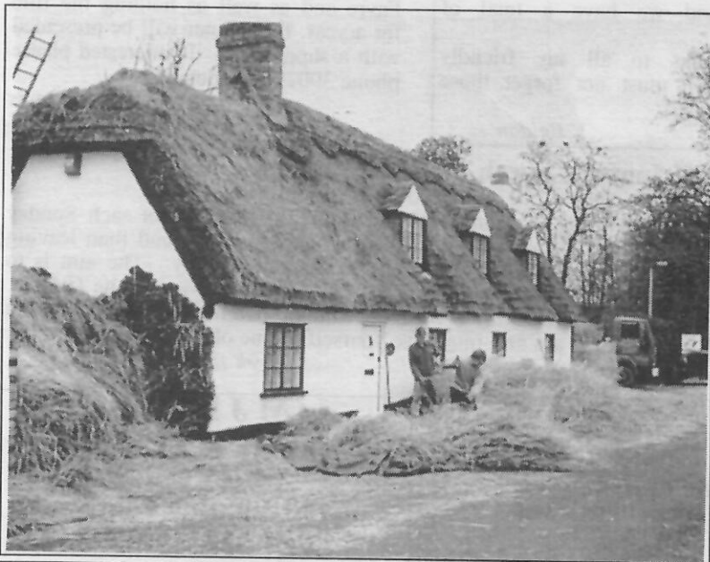
Re-thatching Lilac Cottage in Church Lane
