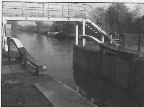
Old lock gates lying at the side of the locks and new ones in place
