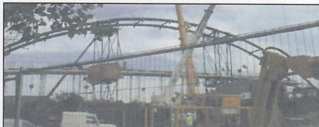
New bridge, standing on the old section of the A10, almost ready to move into position
